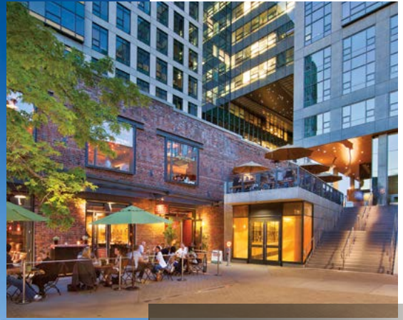
Phase IV of the Amazon.com headquarters included the renovation of the historic Terry Avenue Building, which has been converted into retail space for three restaurants.
